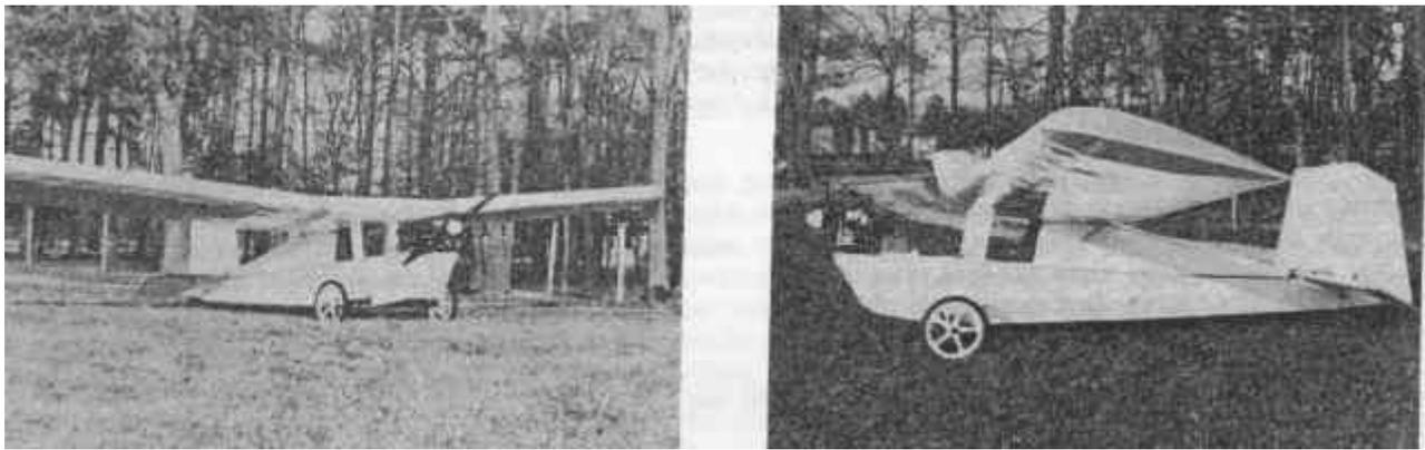
Power is a stock Cuyuna 215 with CPS reduction and a 59 inch Ultra-Prop. Colors are white overall with light blue trim and white wheels to match. This Pup appears to be pretty much per plans except for a unusual modification to the rudder control system. The rudder bar was replaced with pedals, and the cables were routed inside the fuselage—mostly for aesthetic purposes. Rick also added a steerable tailwheel and thinks it helps ground handling on the hard surface runways.
